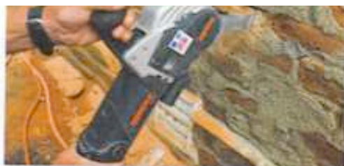
Bricks damaged by unprofessional repointing (mortar replacement) were cut from this wall using a brick-and-mortar saw. Substitute bricks were inserted into the wall so skillfully that the repaired section is indistinguishable from the rest of the existing wall. Photos: courtesy of U.S. Heritage Group
