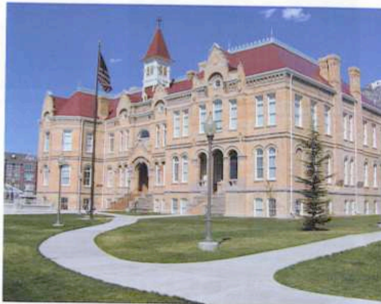
Built in 1892 to house the Brigham Young Academy, this eclectic Victorian building (above) sat empty from the early 1970s until restoration began in 1997. It suffered severe deterioration during the decades it was vacant (left). Damaged bricks were repaired or replaced with historically appropriate salvaged bricks. Photo: courtesy of Child Enterprises
