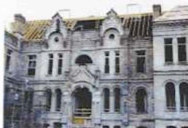
Built in 1892 to house the Brigham Young Academy, this eclectic Victorian building (above) sat empty from the early 1970s until restoration began in 1997. It suffered severe deterioration during the decades it was vacant (left). Damaged bricks were repaired or replaced with historically appropriate salvaged bricks. Photo: courtesy of Child Enterprises
