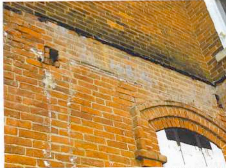
A line of tar marks the edge of a porch roof that was removed from this building. The thick tar cannot be removed efficiently, and the bricks will have to be replaced. Photo: courtesy of U.S. Heritage Group
