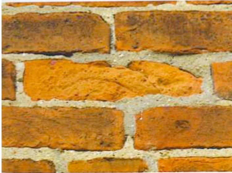
In this case, deterioration is occurring because cement mortar has been used to replace the original lime mortar. The brick is rapidly decaying without the protection of its fire-resistant mortar, which has flaked away. Photo: courtesy of U.S. Heritage Group
